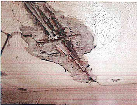
Corroded/Failed Strands over Locker Room
